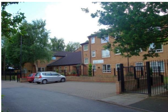
Pavilion Lodge, Stretford
